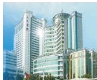
Hubei General Hospital
